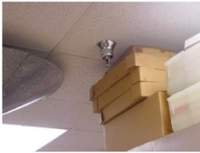
Blocked sprinkler head by storage
